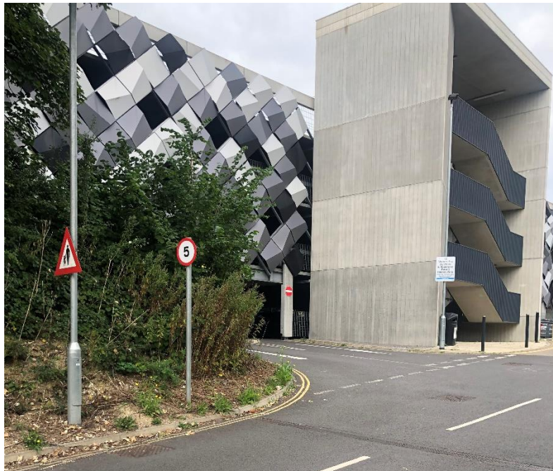
Entrance to P7 Carpark.
